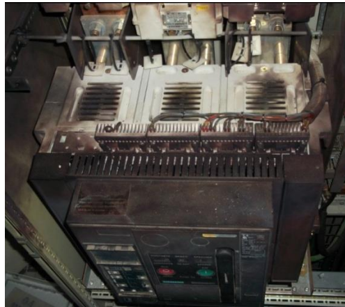
Figure 102. Automatic switch (Source. GDES-COMSA)
