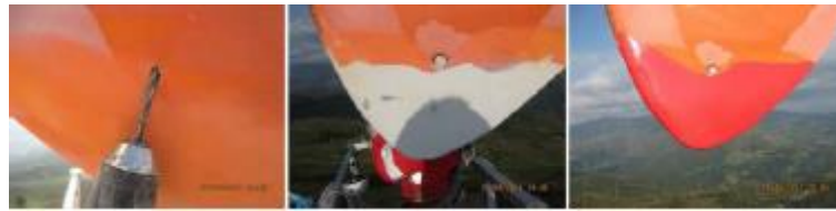
Figure 62. Blade structural repair
