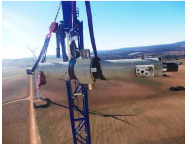
Figure 63. Hydraulic system cylinder deconstruction
