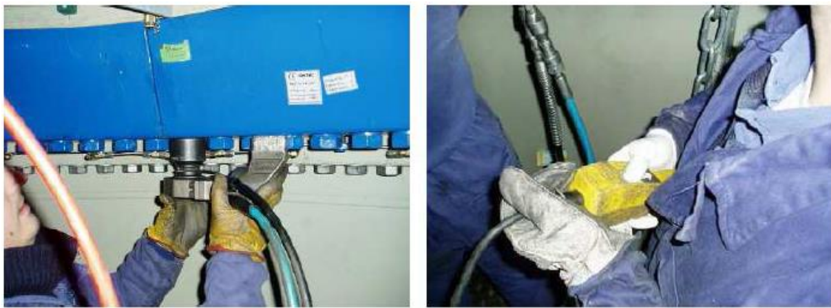
Figure 67. Brakes and clamps replacement
