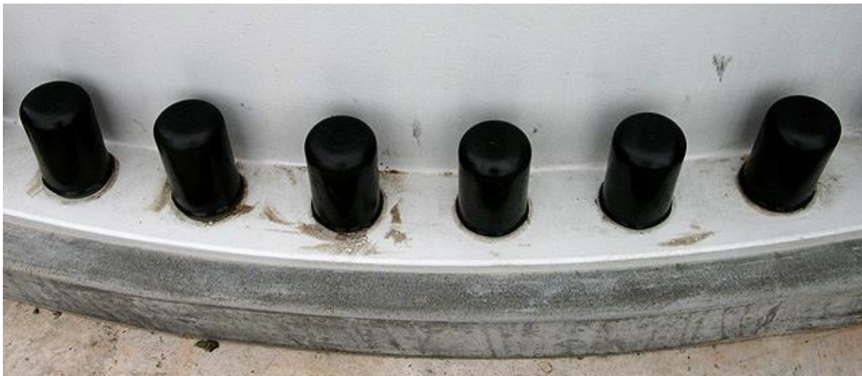
Figure 48. Joint bolt protection caps
