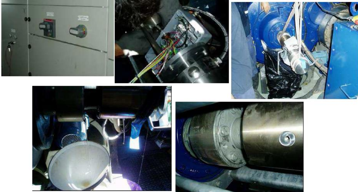
Figure 59. Accumulator removal operation maintenance procedure
