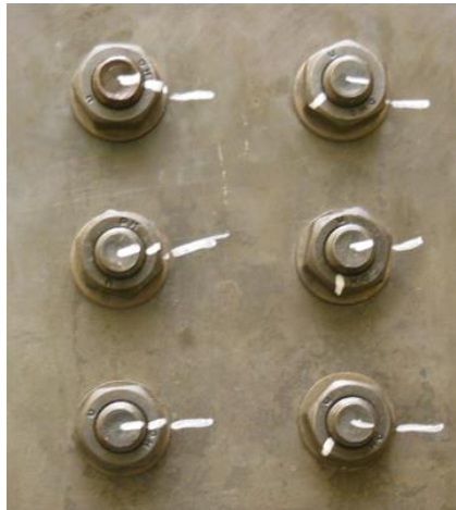
Figure 25. Joint block frame torque checking
