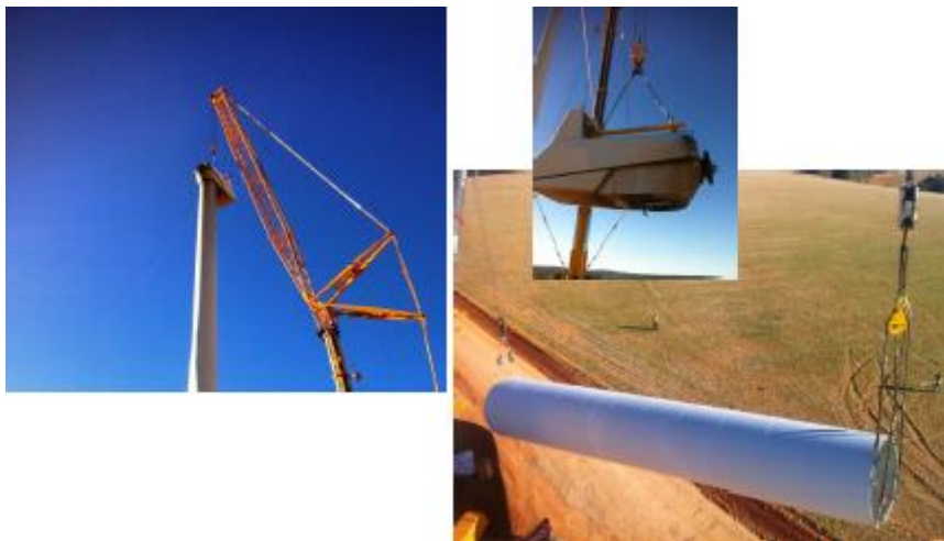
Figure 75. Nacelle and tower removal
