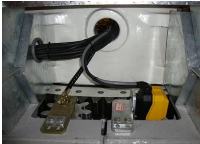
Figure 44. Ring resistor for counting turns
