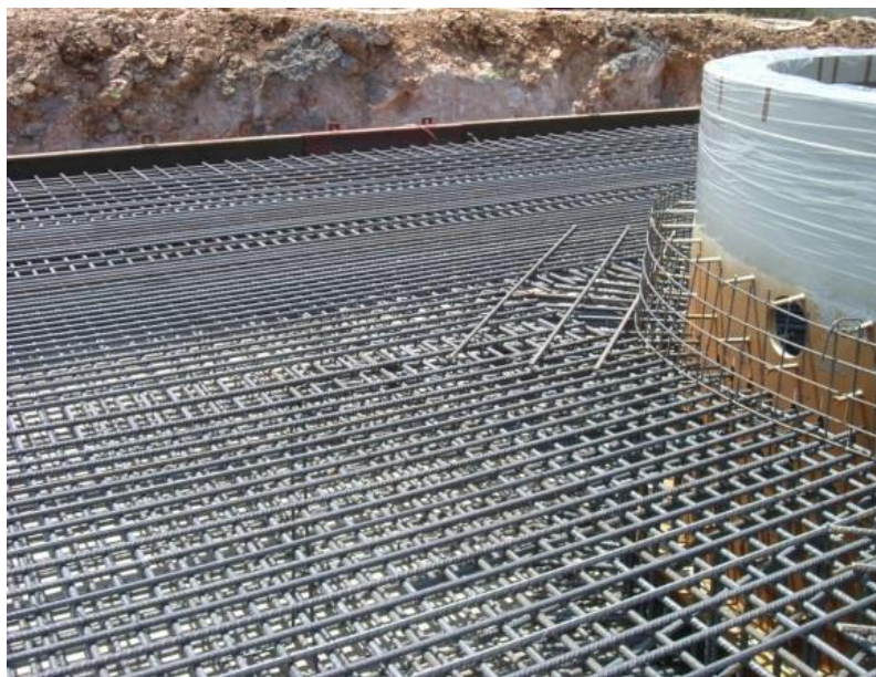
Figure 37. Wind turbine shoe works
