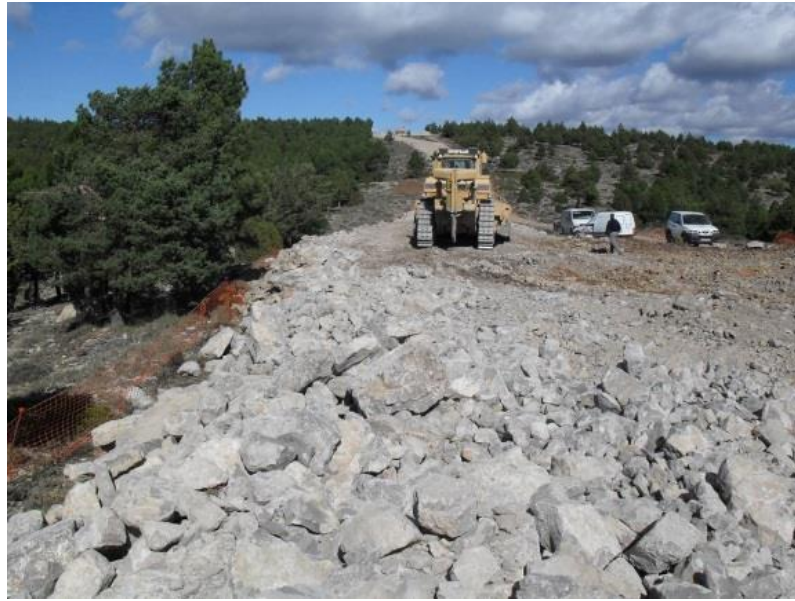
Figure 34. Stone aggregate base for the Wind farma access road
