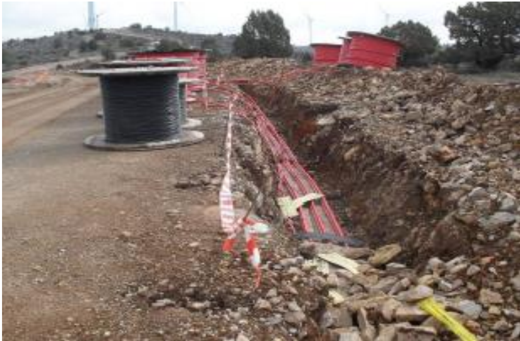
Figure 38. Pipes interconnection between wind turbines
