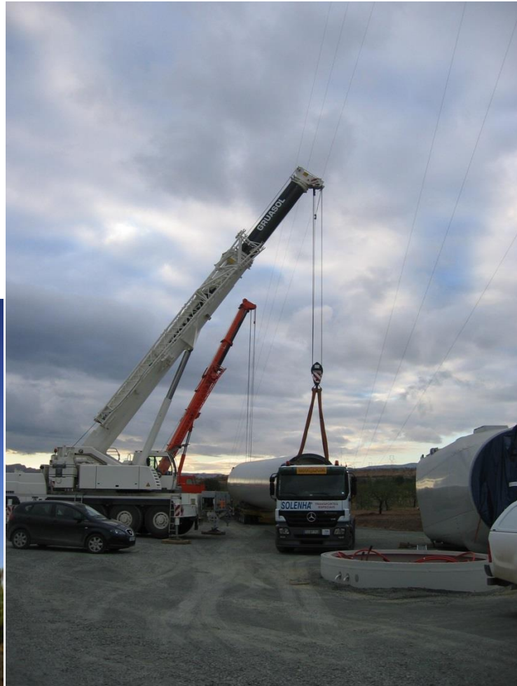
Figure 42. Cranes hoisting the Wind turbine tower
